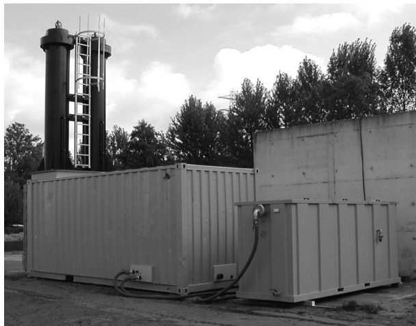
Figure 2 The two reactors of the pilot plant at WWTP Ede, with other equipment in the container and the tank to pre-settle incoming sewage
