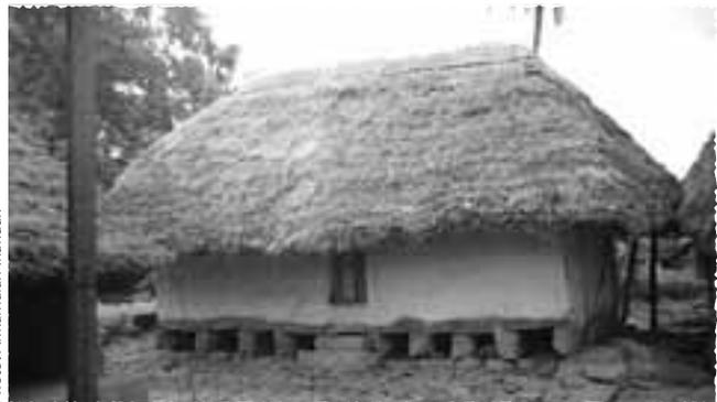
In the hilly tracts of Tamil Nadu (India), a modified out-house structure called seru is becoming more and more popular for storing larger amounts of different grains meant for own consumption, seed or sale. The inner space is divided with mud walls in different compartments, and different grains are stored in separate compartments.
