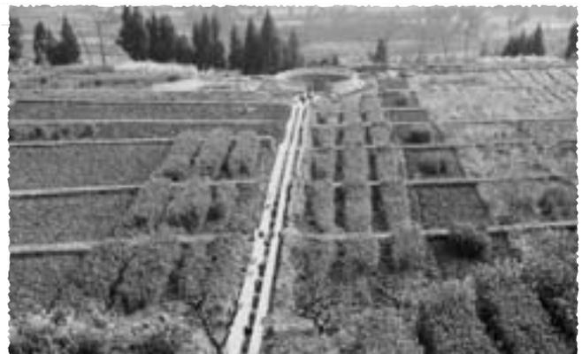
**A ditch diverts water collected on a paved highway to a tank, which provides supplemental irrigation to the crops. The crop in the photo is maize.** Photo: Author.
