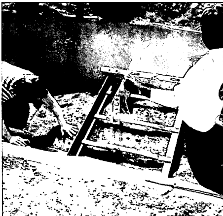
Figure 3.5 The edges of the control section of the flume are formed by steel strips that stay in the concrete. Wire fabric is used as reinforcement of the ramp.
