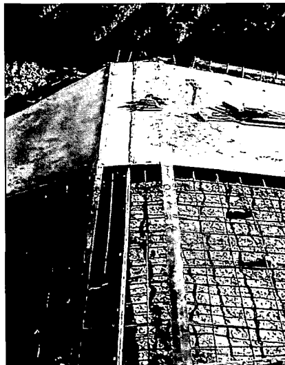
Figure 3.32 The edges of the sill and the ramps consist of an angle iron that remains in the concrete.
