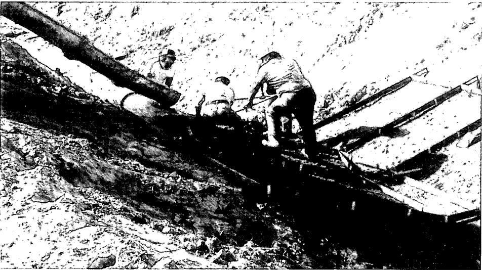
Figure 3.56 Concrete is poured for the downstream toe wall and the diverging transition of a flume with a triangular control section (Arizona).
