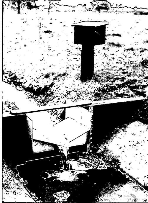
Figure 3.27 Metal broad-crested weir on wooden sheet piling (The Netherlands).
