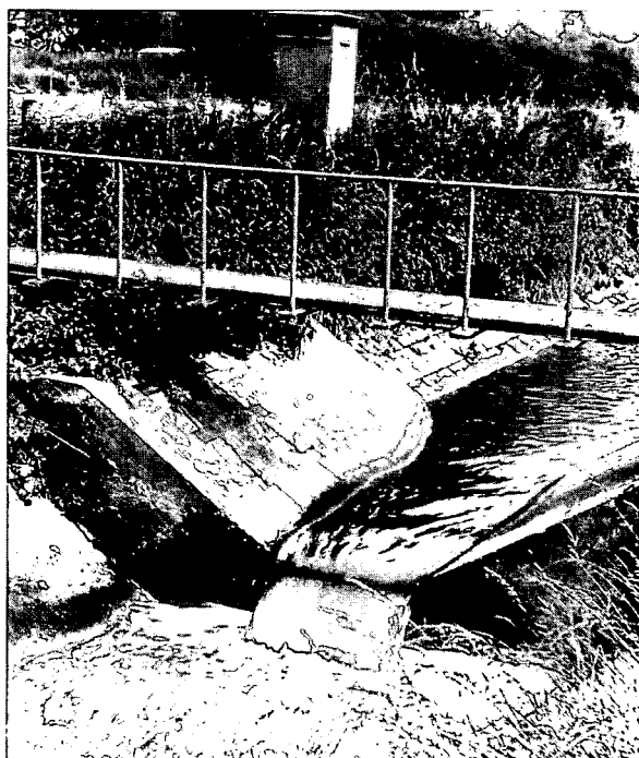
Figure 6.21 If no kinetic energy needs to be recovered, a sudden downstream expansion is adequate (The Netherlands).
