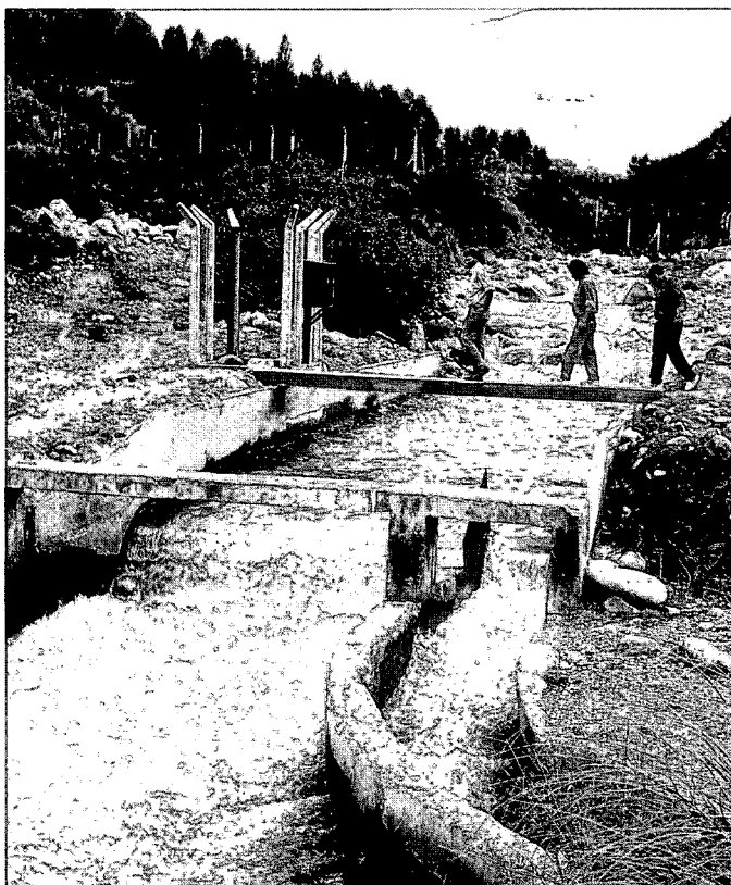
Figure 2.19 The Froude number in the approach channel to the weir was reduced to 0.5 by flattening the hydraulic gradient. A fixed division board is used to divert flow for irrigation (Argentina).
