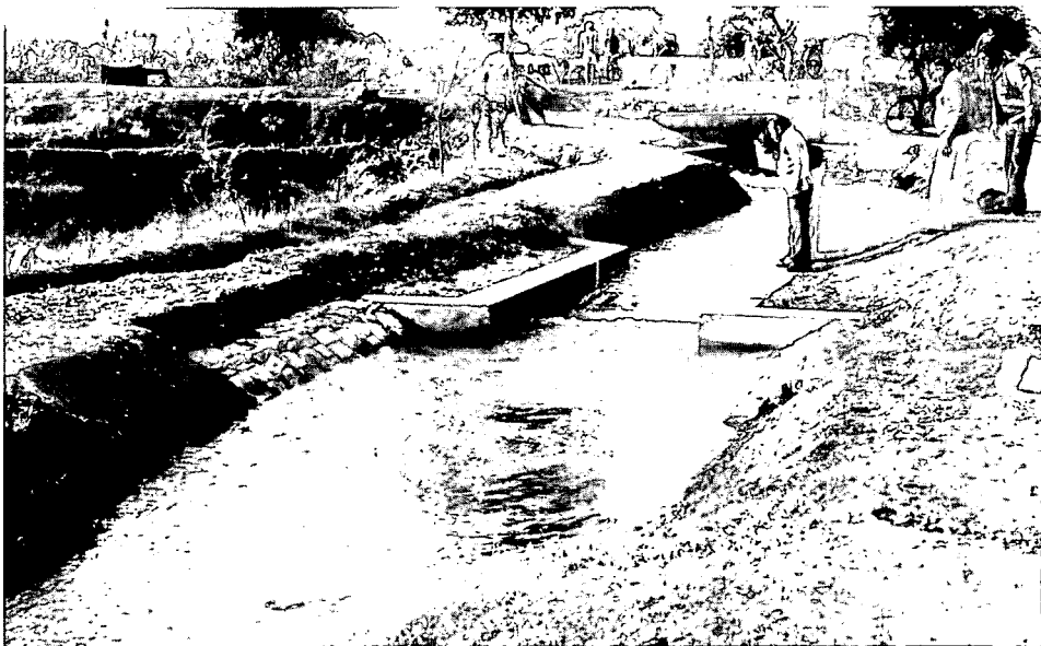
Figure 3.23 Flow measuring structure with a rectangular control section in an earthen canal (India).
