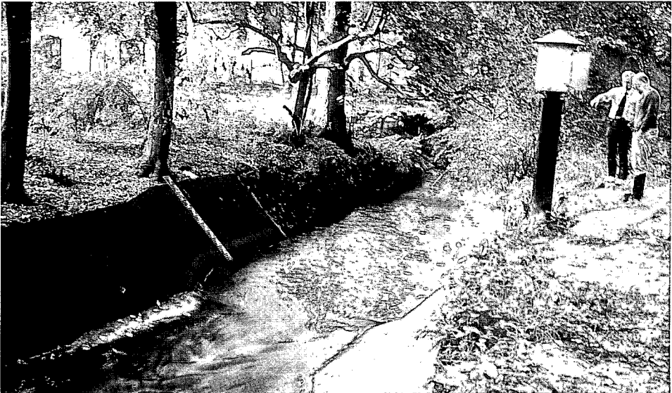
Figure 3.1 This marine plywood flume blends unobtrusively with its environment (The Netherlands).
