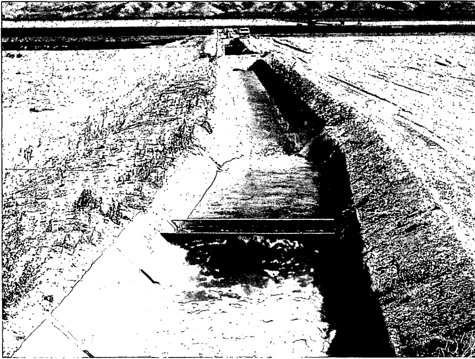
Figure 2.18 A wave suppressor stills the upstream water level to improve the head-measurement accuracy upstream from a broad-crested weir (Arizona).
