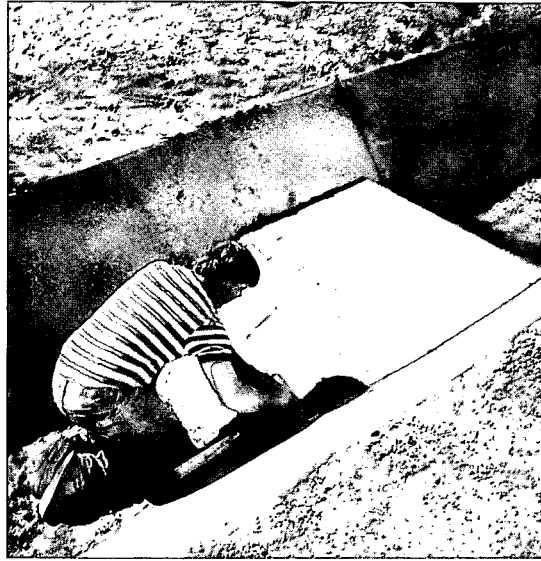
Figure 3.7 The ramp can be hand-troweled into place.
