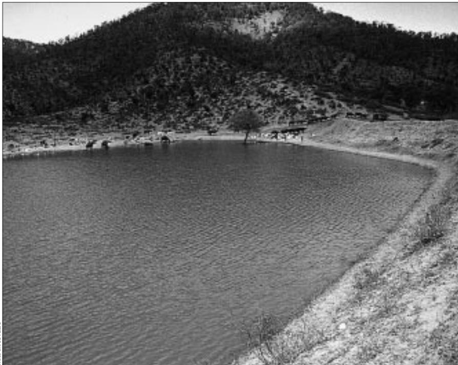
*The Johad is a structure bound on three sides by the natural slopes of the hill. The fourth side, a mud wall – usually semi-circular in form – holds back the monsoon run-off.*
