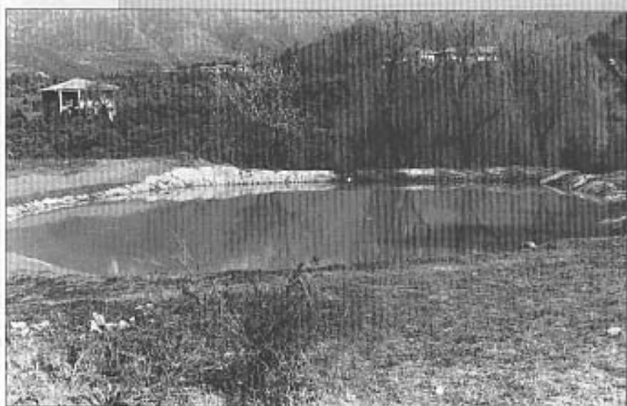
In Himachal Pradesh, India, poly-lined tanks are useful and cost-effective for water harvesting.
