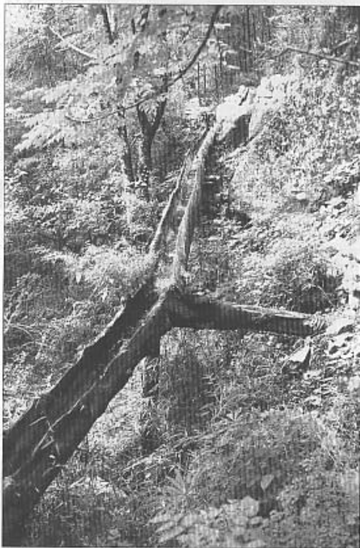
A wooden aqueduct in the irrigation channel.
