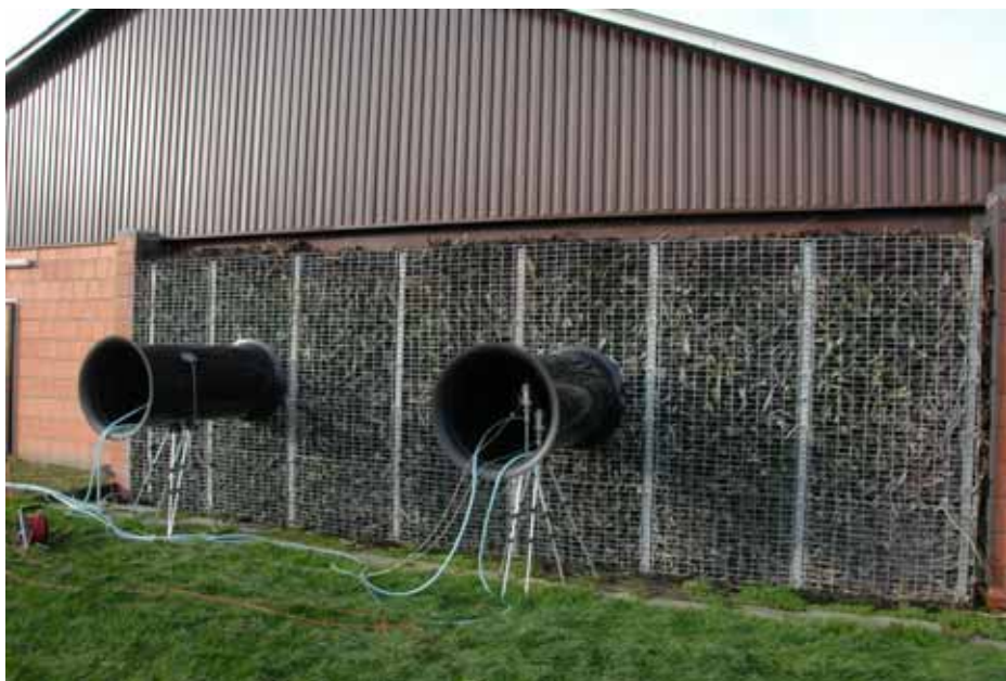
Figure 5.3 Air scrubber next to an animal house with a large surface of the outgoing air. Air is sampled inside tubes placed on the last layer of the scrubber to prevent wind influences
