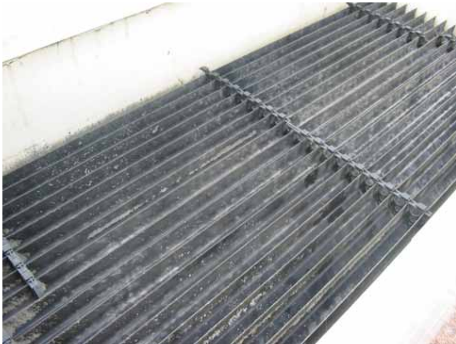
Figure 5.2 Droplet remover of a combined air scrubber where the cleaned air is coming out
