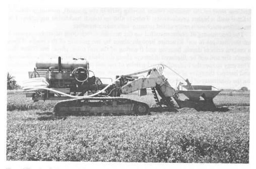
Figure 3 Trencher drainage machine, steep chain type, installing corrugated pvc pipe with gravel surround in Egypt. Note water tank for wetting chain and trench box sides to avoid sticking of clay.
