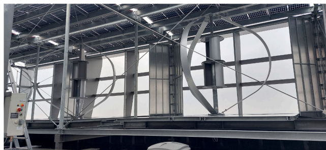
Fig. 4. PowerNest turbines integrated with solar panels (the picture was taken by the first author).
