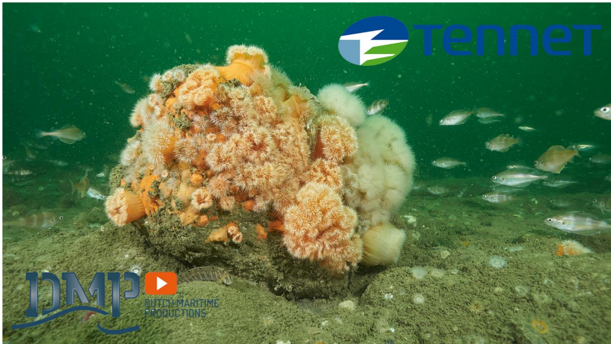
Figure 8. Example of armour layer rock coverage after 2 years of deployment at cable crossing of Hollandse Kust Zuid export cable (Source: Dutch Maritime Productions).
