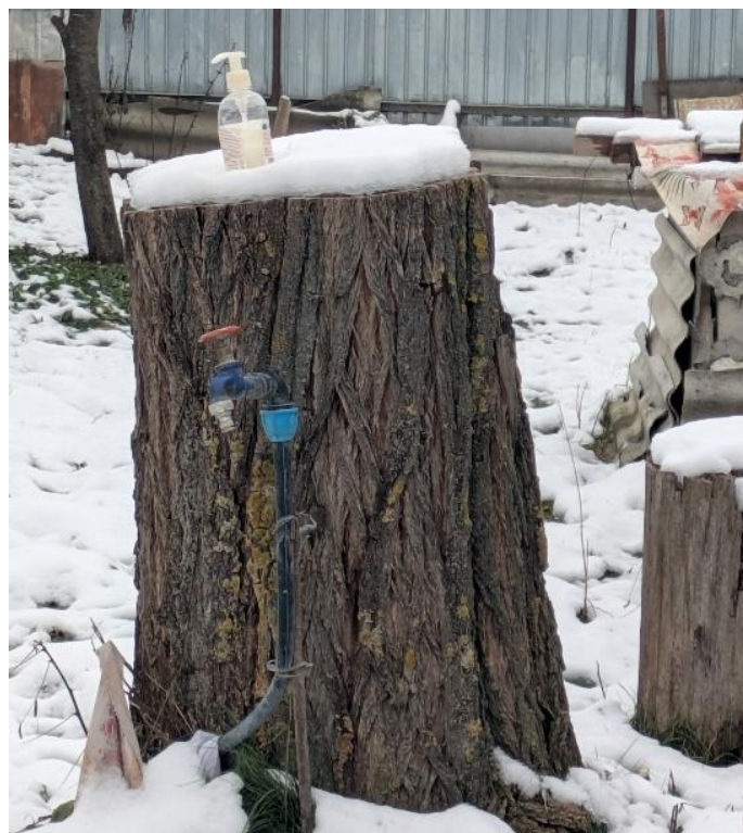
Figure 14: Outdoor water pump
