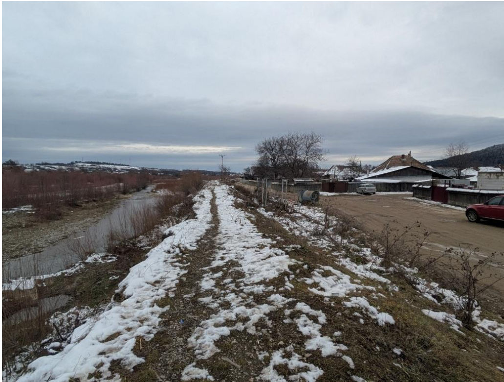
Figure 4: The land is at risk of flooding from the Cracău River
