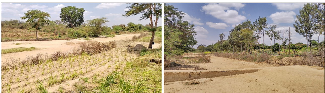
Figure 3. Planting of Napier grass along the Enguli River for bank protection (left), and a sand dam constructed near Kasikeu with restored sand levels (right) (photos taken September 2023, credit: Duker)
