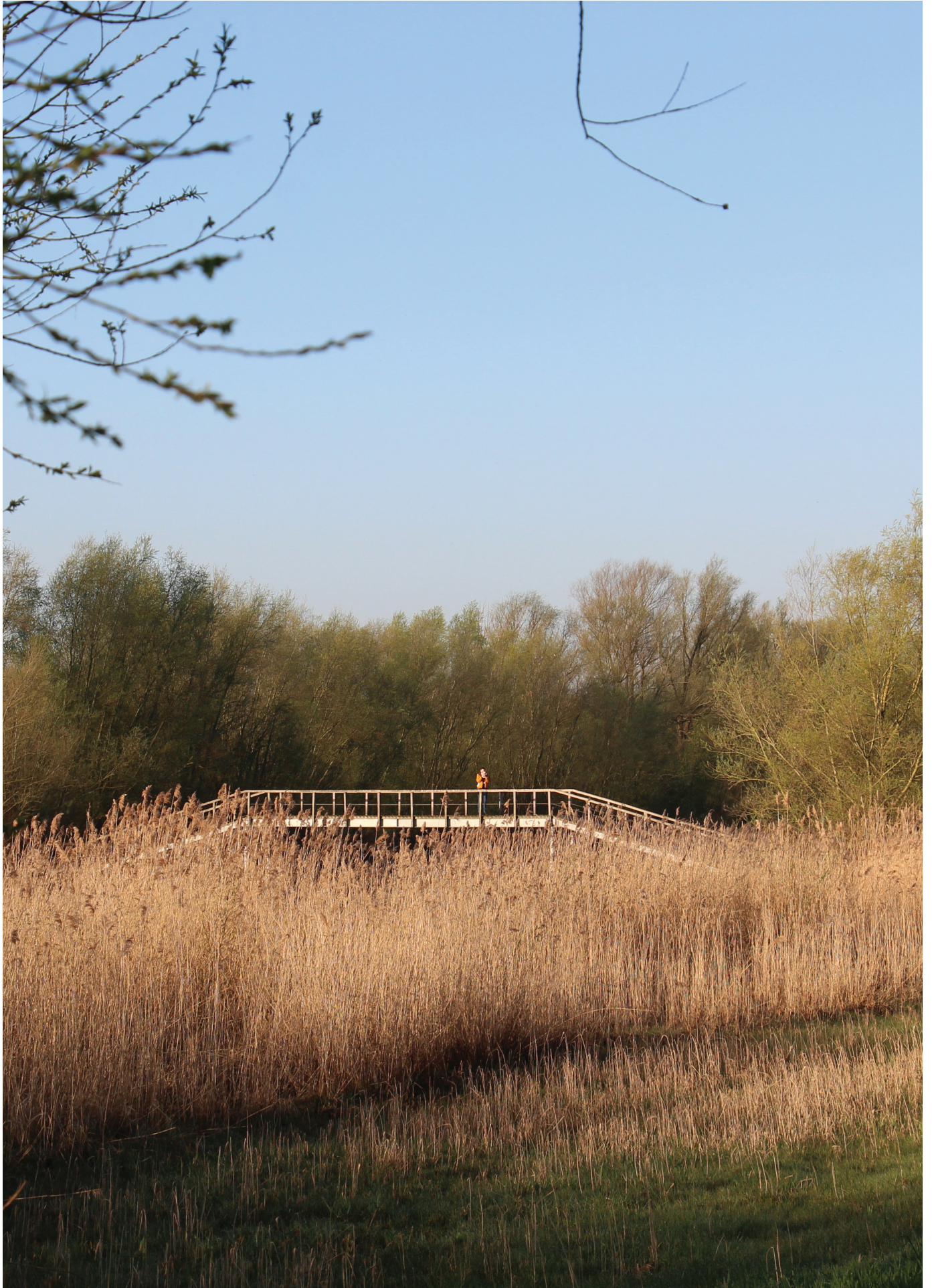
The bridge over the secondary channel.
