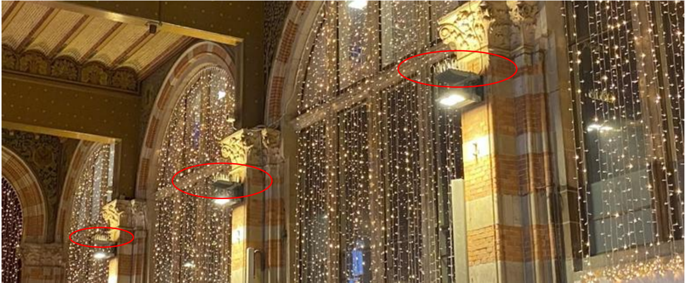
Picture 11: Spikes to deter pigeons presence on lamps in the main entrance hall
