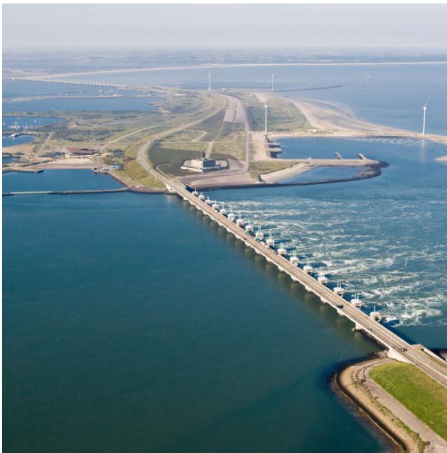
Figure 3: The Eastern Scheldt Barrier. This barrier was constructed as a semi-permeable dam with sluice gates installed after ecological concerns were addressed for the first time in Dutch coastal flooding and water management policy in the 1970s (Meijerink, 2005; Watersnoodmuseum, n.d.)
