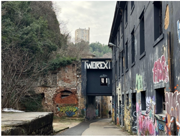
Figure 24. Hartera building. Note. Photograph by the author.
