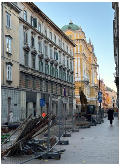
Figure 14. Construction work in the city centre 1. Note. Photograph by the author.
