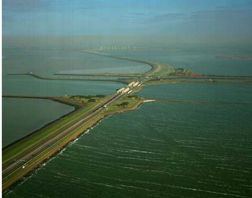
Figure 1. One of the existing discharge facilities in the closure dam. The lake is to the right and the Wadden Sea to the left
