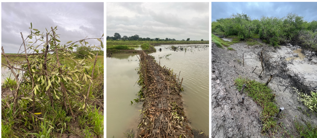
Figure 7 – Avicennia spp. used to build a fence in the rice fields; to repair a dike; to strengthen dam.
