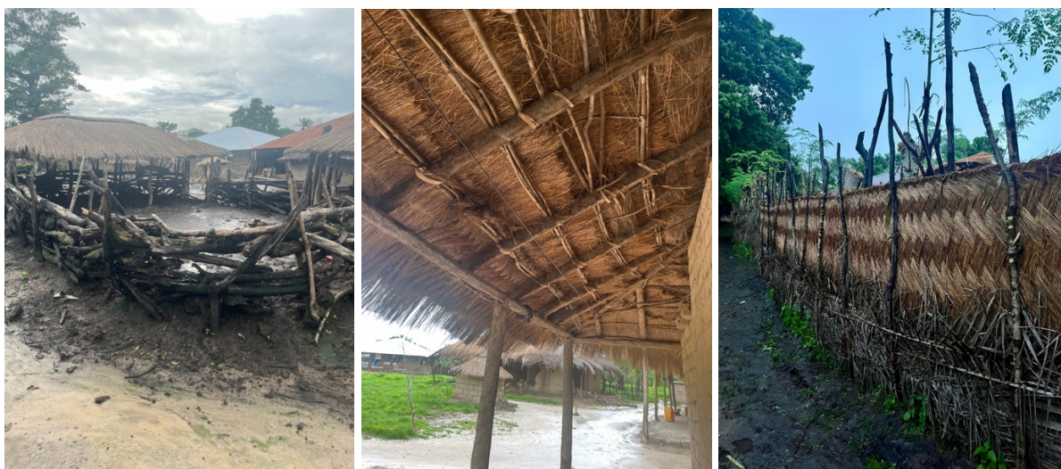
Figure 8 - Avicennia spp. for cow's fences; Rhizophora spp. for house structure; Laguncularia spp. for house fences
