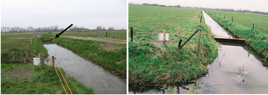
Figure 4 View from position F1 (left) and position F2 (right) as indicated in Figure 3.
