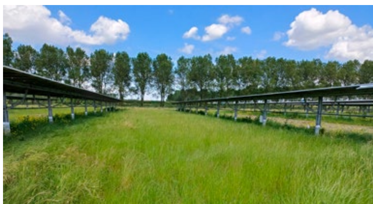
Examples of agrivoltaics Systems. Left: Solar panels over pear orchards (photo W. Eerenstein). Right: Rows of solar panels with space for cultivation in between. Top right: Vertically placed panels (photo WUR). Bottom right: Panels that follow the sun (tracking systems) (photo W. Eerenstein).
