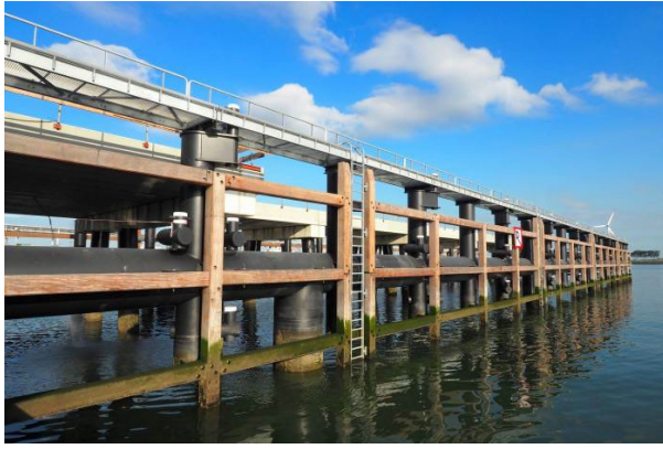
Figure 8 Fender in Rotterdam (NL). (Photo www.houtindegww.nl )
