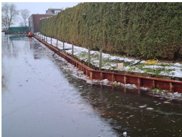
Figure 3 Revetment in Stolwijk (NL). (Photo www.houtindegww.nl )
