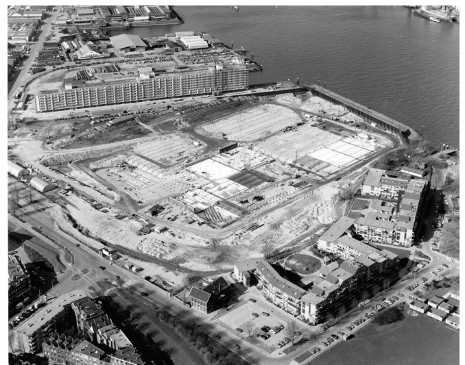
Figure 116 Building of the AWZI (Hofmeester and Dijkstra, 1984).
