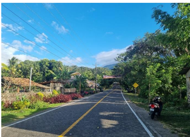
Figure 9: New concrete road connecting Santa Cruz and Balgüe on Ometepe island, source: Author
