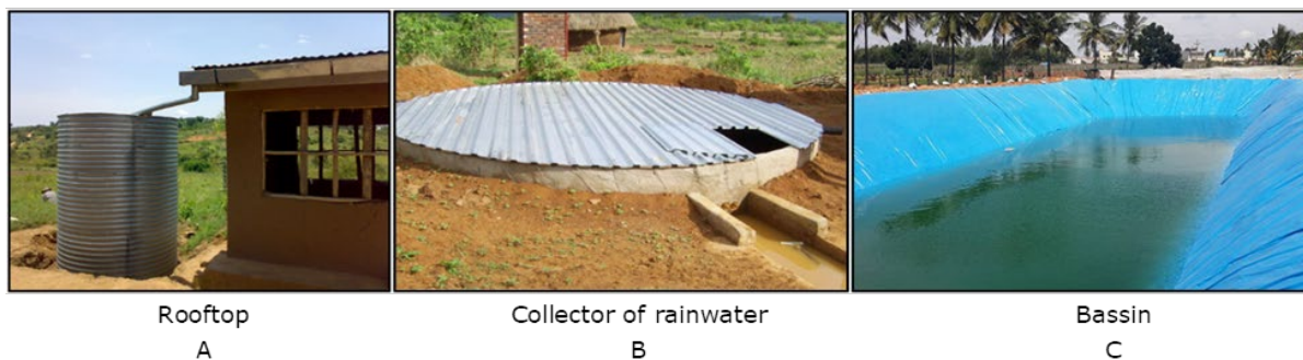
Figure 4. Three different techniques of rainwater harvesting for agricultural production. Source: (Linderhof et al., 2022).
