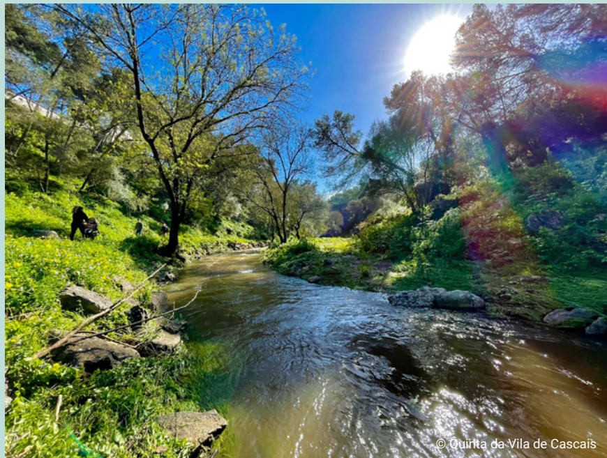
Figure 13.1 Riverbed restoration project, Cascais
