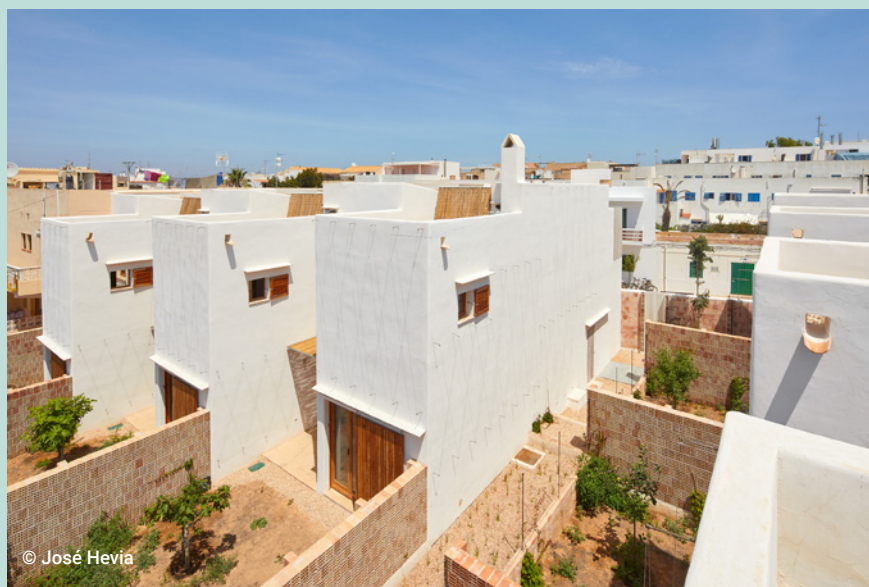
Figure 5.1 Posidonia project, Balearic Islands, Spain
