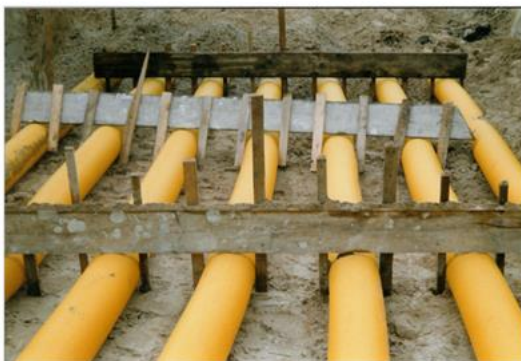
Figure 5.2.2: Installation of underground tubes used as an air inlet (@WUR)
