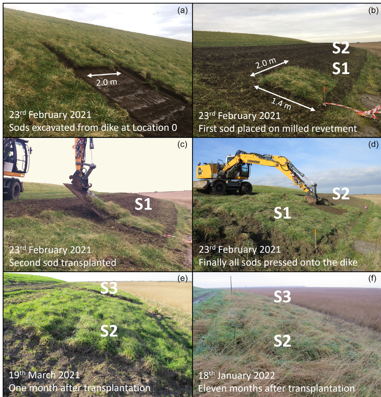
FIGURE 3 Grass sod transplantation technique. Grass sods excavated at Location 0 (a) and transplanted to experimental plots at the waterside dike slope (plot S1 in b, c, d and S2 in e, f). SodS were placed on the milled dike revetment (b, c) and pressed (d) to enhance firm connection with the dike. (e, f) Impression of sods plots after transplantation. Locations in Figure 1.
