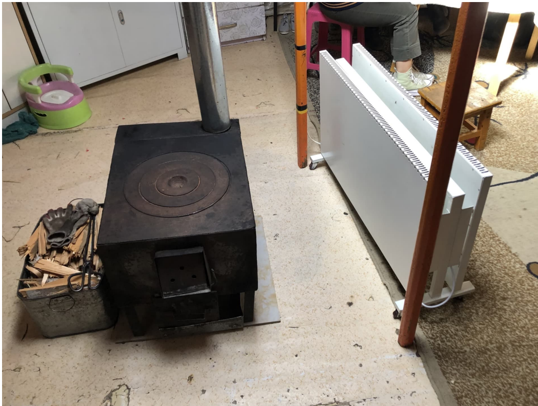
Figure 1: A traditional coal stove standing next to an electric heater, in the ger of a household participating in an electrification project of the startup URECA. To the left of the stove, there is a metal container with the wood used to light the coal stove, and gloves to handle the coal and wood. (April 2023)
