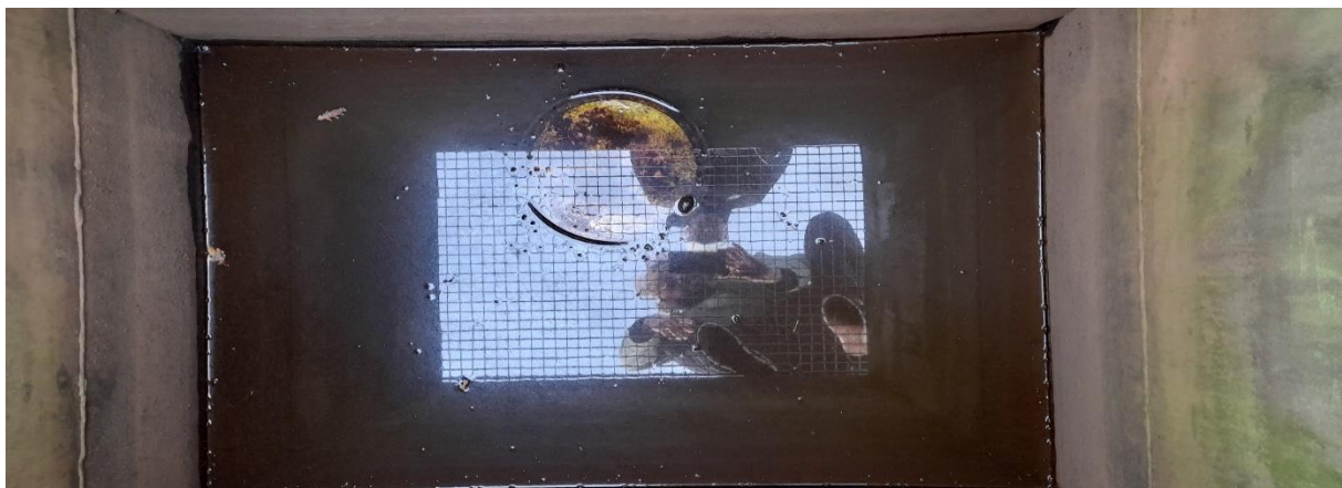
Figure 8: Stagnant water in a 'De Wit' fish passage because it is closed, whilst there is no apparent reason for closing it as there is a lot of water flowing over the weir next to it (Observation report).
