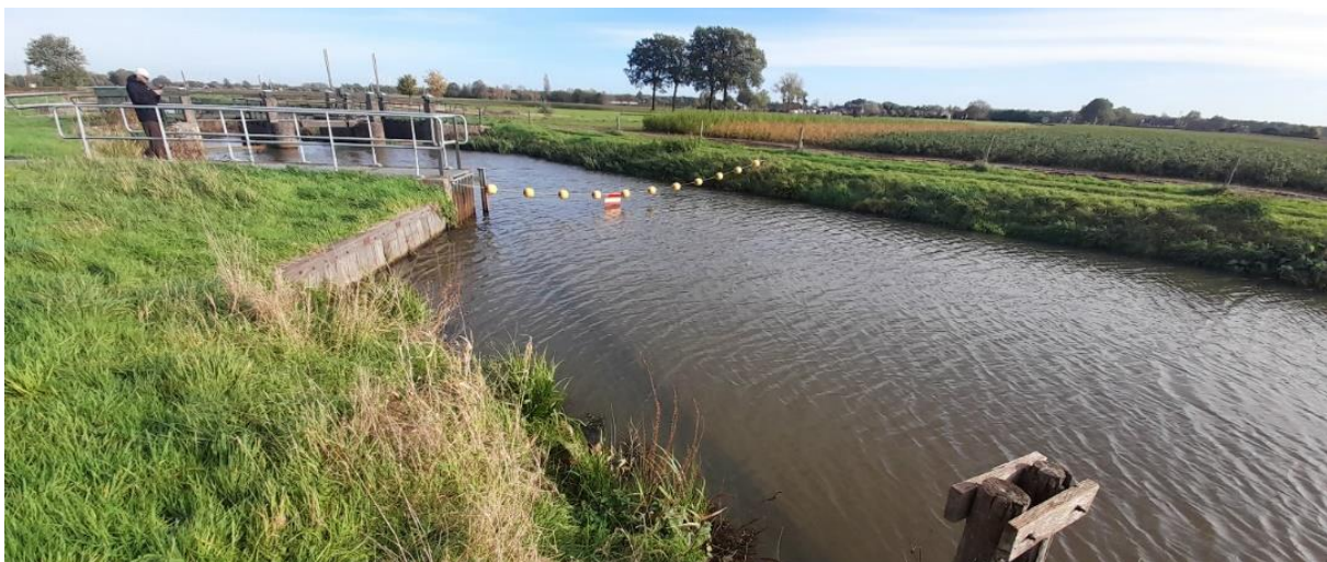
Figure 10: The wooden beam in front of a technical fish passage that lost its function of preventing debris from entering the fish passage, which resulted in a clogging at the entrance of the fish passage, inhibiting fish migration (Observation report).
