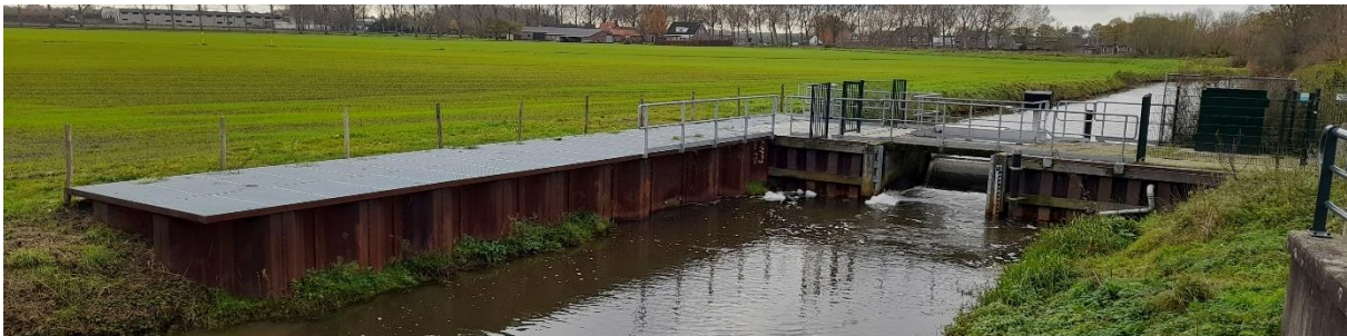
Figure 6: A technical 'De Wit' fish passage that does not take up a lot of space, next to the land of a farmer (Observation report).
