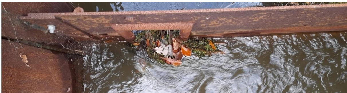
Figure 9: A technical 'Vertical Slots' fish passage with debris stuck in one of the slots that the maintenance employee did not want to clean (Observation report).
