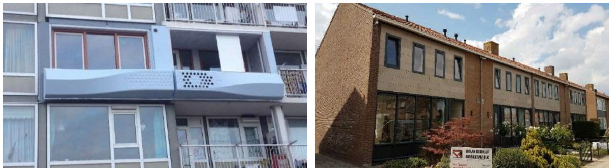
Figure 21 Biocomposite facade panels; on the left containing an air-to-heat pump; on the right as cladding of the 1st floor. Photos: NPSP.
