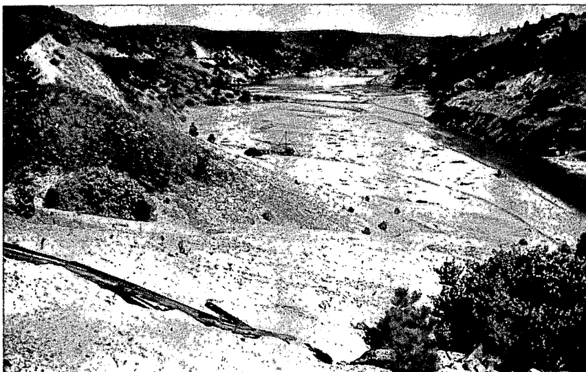
Figure 3. Downstream view of the 10 years old, 0.8 km long, Spring Creek Delta in Keswick Reservoir. The thickness of highly acidic sandy alluvium was locally over 12 m
