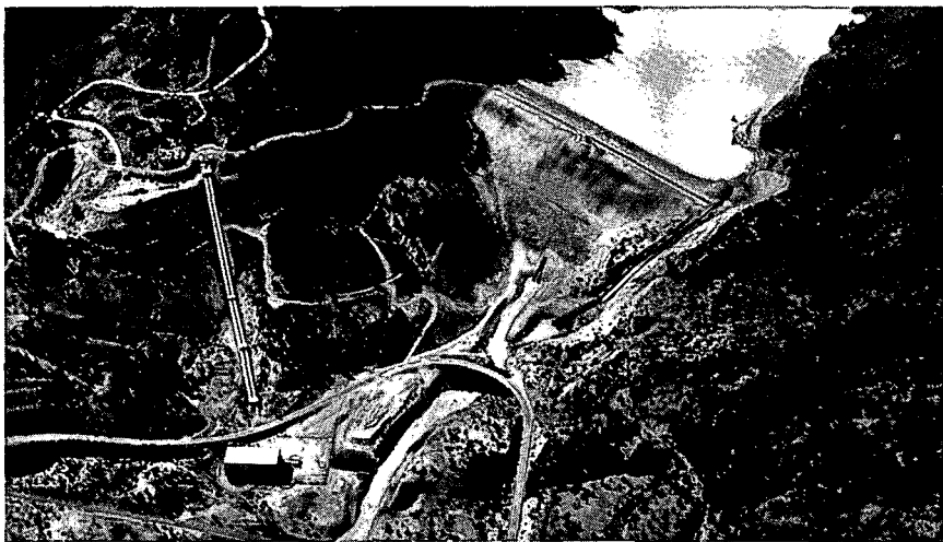
Figure 5. An upstream view of the 60 m high Spring Creek Debris Dam during rainy season (During summer-fall seasons the reservoir is nearly dry)
