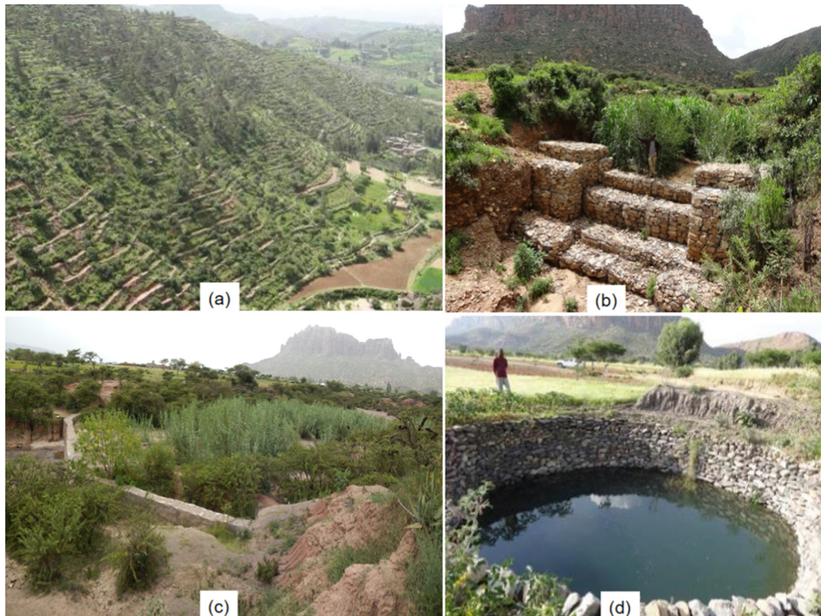
Fig. 4. Examples of the interventions at different parts of the landscapes: (a) SWC at upper sections of the landscapes, (b) gabion check-dam integrated with biological measures, (c) sand dams for sediment and groundwater storage and recharge, and (d) shallow groundwater wells developed at lower parts of the landscapes.
