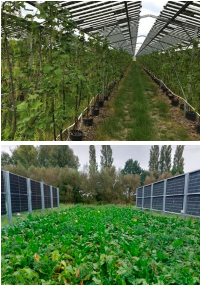
Figure 1 Above: red currants grown under solar panels; the panels are semi-transparent to ensure that sufficient light reaches the fruit (photo: Frank de Ruijter). Below: vertical panels, in between which crops can be grown (photo: Thomas Reher). The panels are double-sided (bifacial) and can generate electricity on both sides. The rows will be installed in a north-south alignment and the panels will then produce the most power in the morning on the east side and in the afternoon on the west side.
