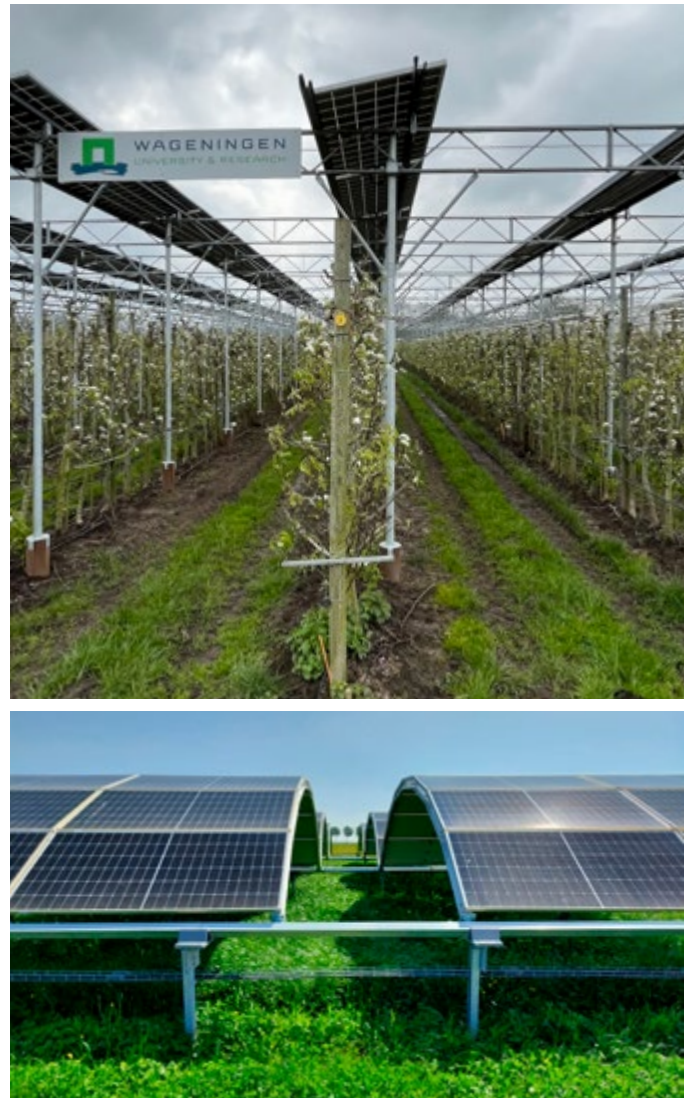
Figure 2 Above: solar panels over pears (Groenleven system; photo: Frank de Ruijter). Below: Mobile solar arches from GOLDBECK SOLAR/Solarvation over grass/clover (photo: Jan-Rinze van der Schoot).
