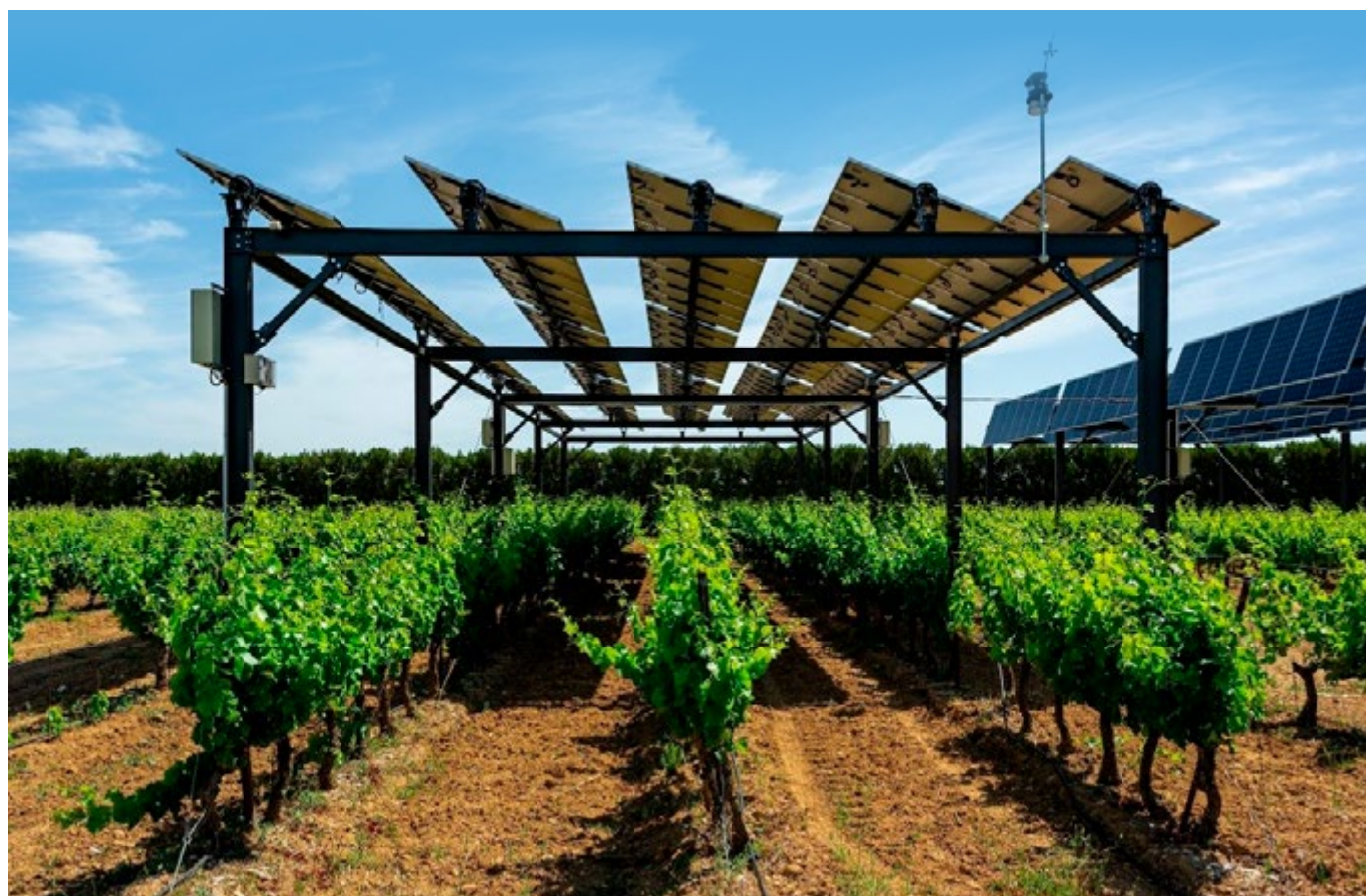
Figure 3 Movable panels over grapes in Piolenc, southern France (photo: Sun'Agri 8 )
