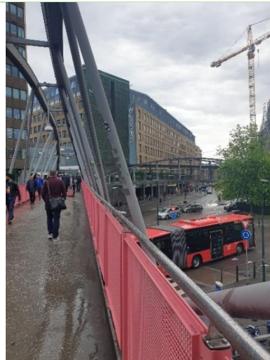
Figure 5.4: Pedestrian bridges in front of the central train station Oslo
