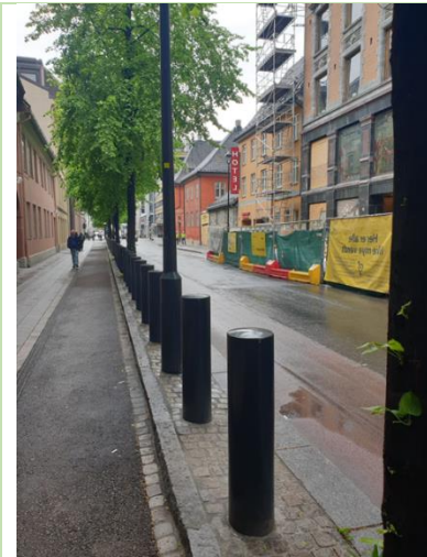
Figure 5.3: Bollards that separate walkways from motorways
