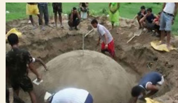
Photo 1: construction of a household biodigester in Nepal (credits SNV Nepal)
