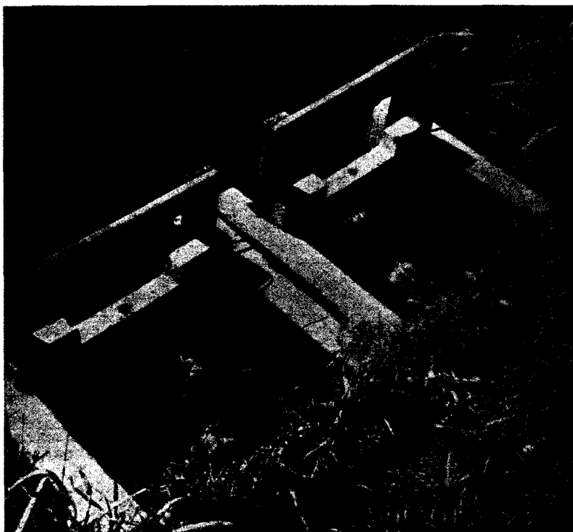
Photograph 6. A double weir in a supply ditch.
