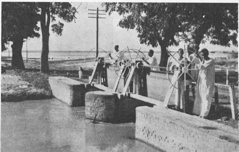
Photo 6. A water control point
