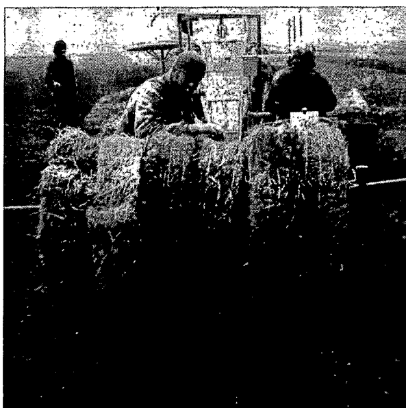
Fig.7. Covering pipes with flax strip.
