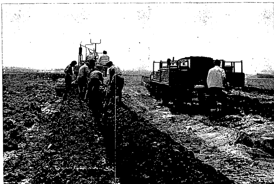
Fig.4. Mechanized drainage with clay pipes. The pipes are taken from the trailer and laid on a platform. Two workmen apply the peat fibre.
