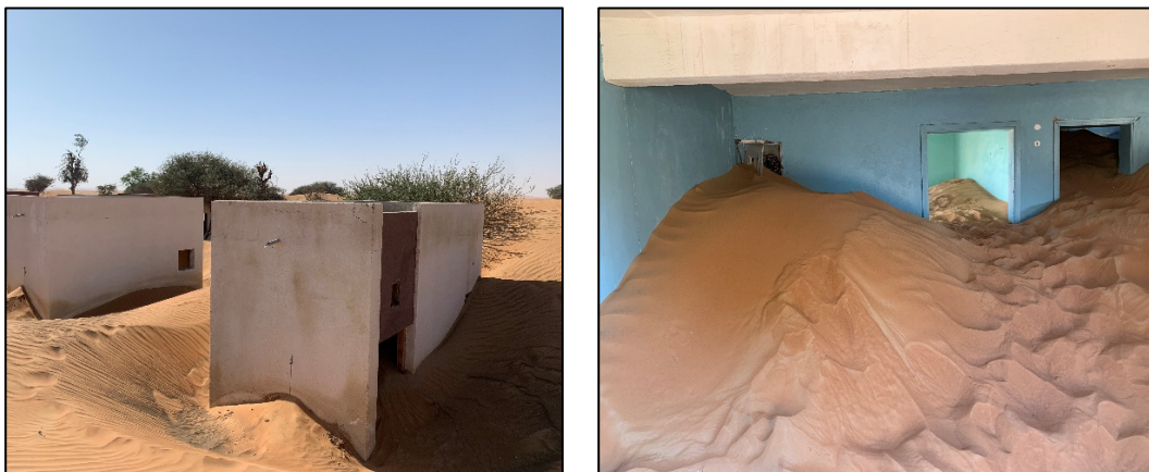
Figure 11. Sand accumulations between two buildings (left) and inside a dwelling (right) in Al-Madam, UAE (photos: M. Sherzad).
