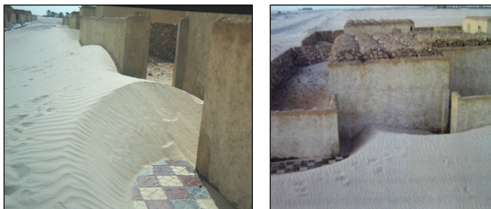
Figure 3. Sand encroachment on a new housing project in the region of El-Oued Souf, Algeria. (Photos: M. Sherzad).
