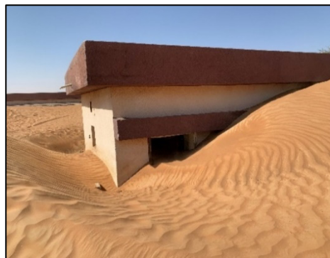
Figure 2. Dwelling covered by sand in Al-Madam, UAE. (Photo: M. Sherzad).
