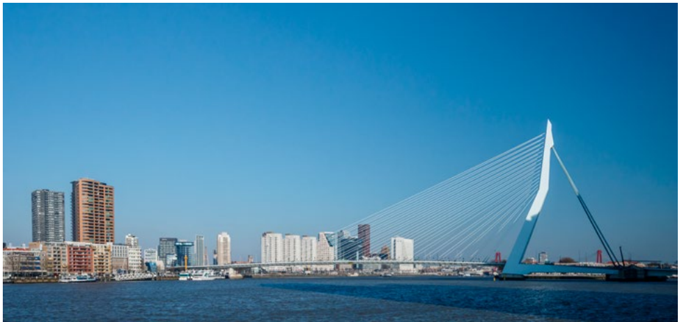
Figure 1. Illustration of Harbor bridge of Rotterdam
