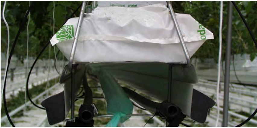
Figure 9 An example of the pipes (light green) used for CO 2 distribution from flue gases, obtained through personal communication with Frank Kempkes. The size of these pipes corresponds to the concentration of CO 2 being distributed, which is 8% in the case of CHP flue gases.
