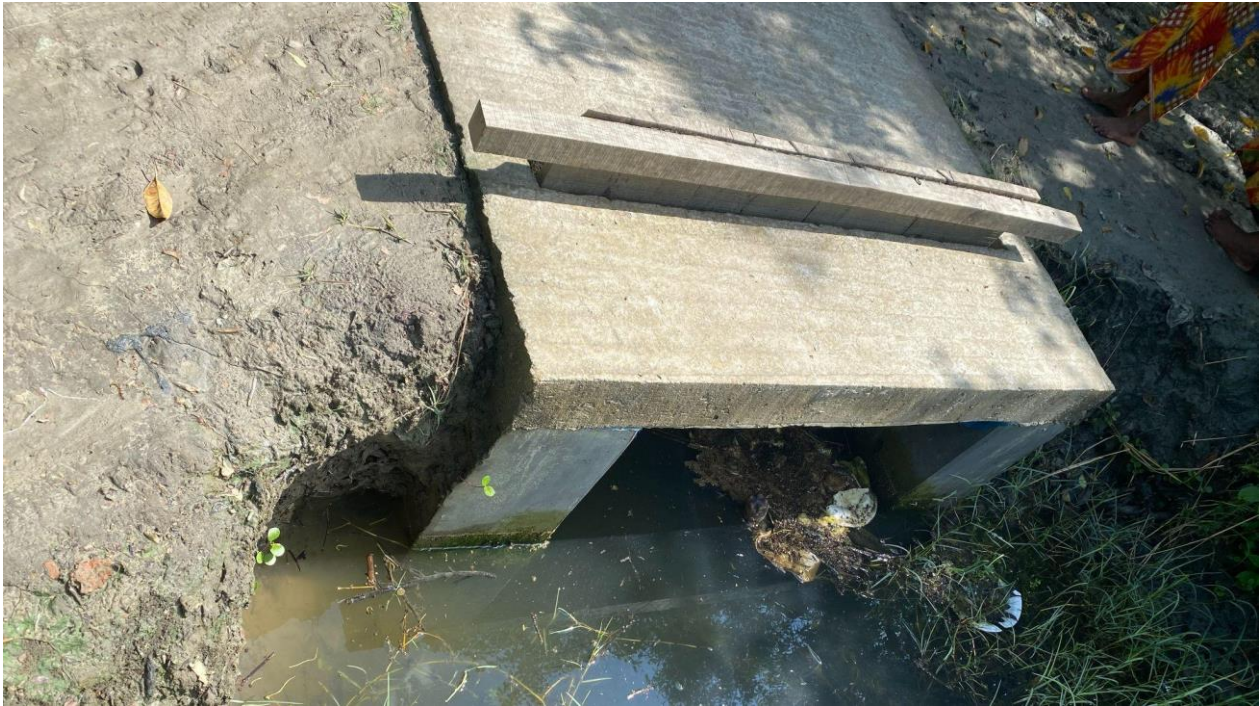
Figure 27 Sluice gate between the re-excavated canal and the Goater Khal.
