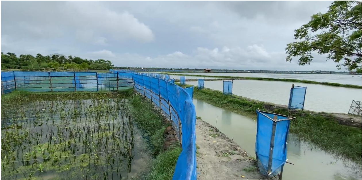
Figure 31 Part of the re-excavated canal, with on the left the mangrove nursery in the micro-watershed, surrounded by shrimp ponds.
