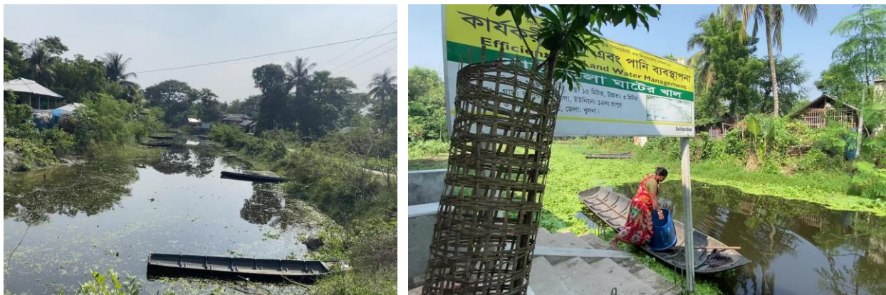
Figure 5 Left: The re-excavated canal under Pilot 1, used for transportation, Right: The pavement that connects the re-excavated canal to the vegetable collection centre.
