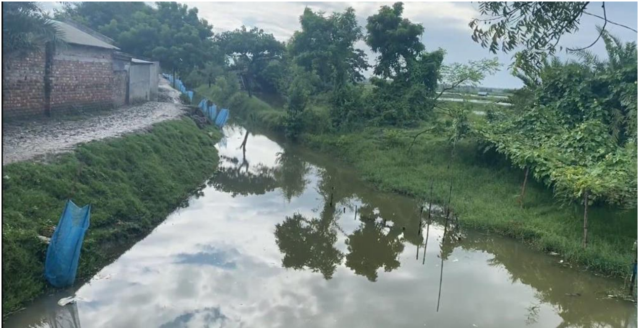
Figure 23 The deeper part of the re-excavated canal and farmers cultivating vegetables around the canal. The blue protects the mangrove trees from being eaten by livestock. On the left side of the canal, a reconstructed road is shown.
