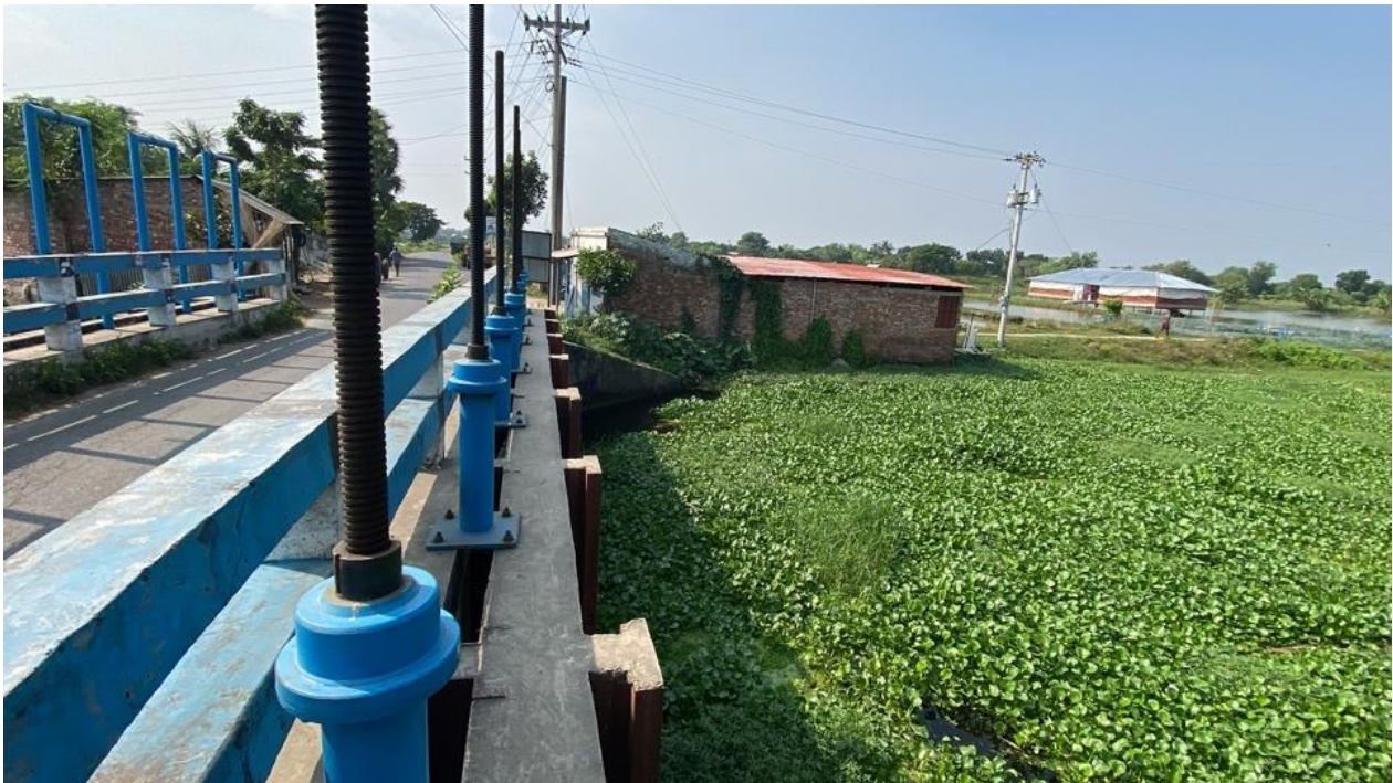
Figure 7 Sluice gate connecting the '80 feet canal' with the Shalua river.
