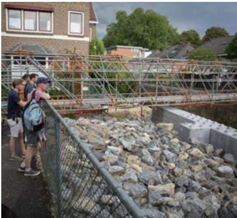
The temporary bridge over the Geul in Valkenburg
