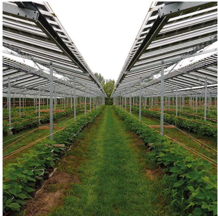
Fig. 3. Mixed-production Solar Power Plant ‘Babberich Agri-PV’ in the east of the Netherlands. Left: the high number of economic properties in this case illustrates the focus on economic considerations. Right: Raspberries grow in an improved micro-climate and the panels protect the fruit from extreme weather conditions. The semi-transparent panels generate electricity and leave enough solar irradiation for the growth of the raspberries.
