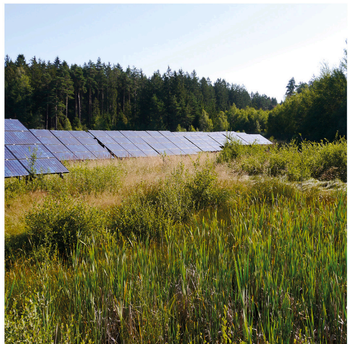
Fig. 4. Nature-inclusive Solar Power Plant Hemau in Germany, near Regensburg. Left: Hemau illustrates some attention to landscape and economic considerations, but most measures are taken for nature. The area covered by PV panels is relatively low because of the high row-to-row distance and areas kept free of PV panels to preserve and improve ecological conditions. Right: wet habitats have been created within the SPP.
