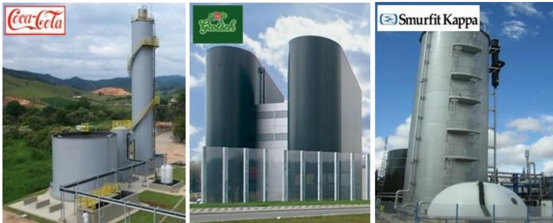
Figure 6 Examples of water treatment systems based on the Paques technology.
