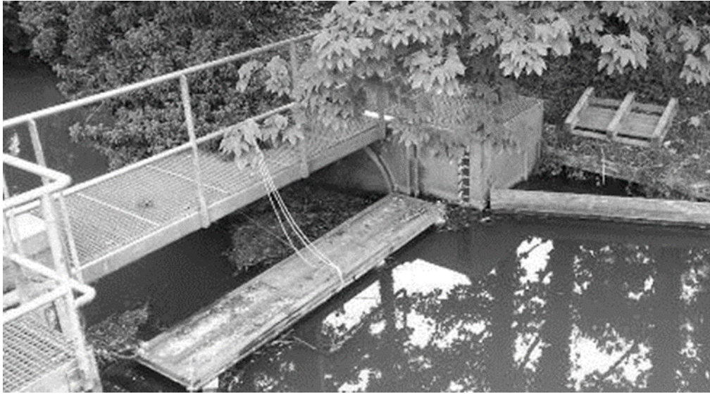
Figure 3.6. Photo of a floating PIT-loop at a weir site.
