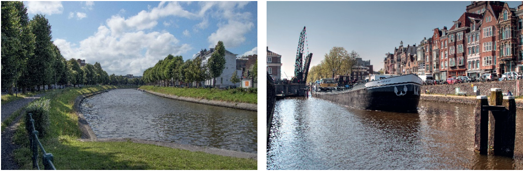
Figure 4.2: Most canals and canalized rivers have vertical quay walls (right, Schippergracht in Amsterdam), some have sloping banks with hard bank protection (left, Coupure in Ghent).
