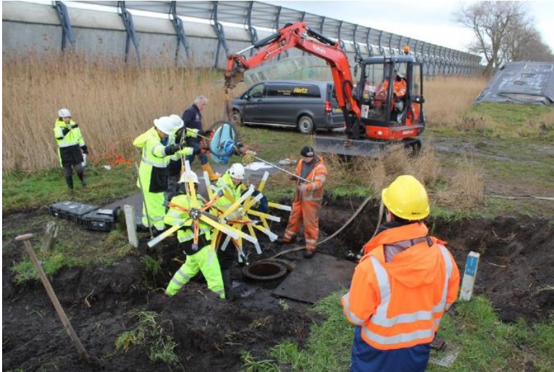
Figure 2: Field team during Pipediver's insertion procedure.
