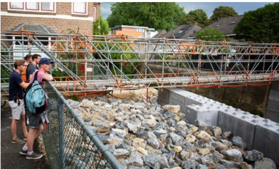
The emergency bridge over the Geul • Photo Jeroen Poelert
